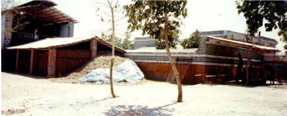
DESI Power plant at Orchha supplies power to a hand made paper factory
